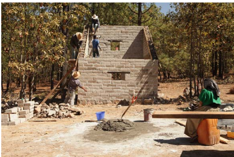
Constructing the solar oven ~ Photo © Gerardo Ruiz Smith 2014
